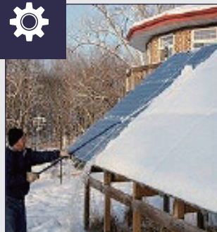
Solar Power Plant located in heavy snow area in winter
